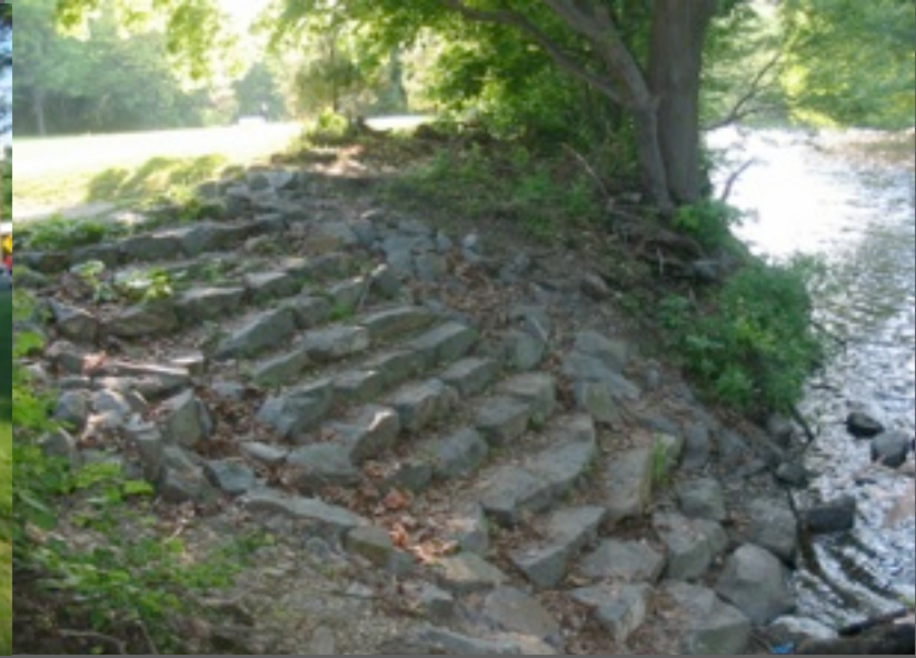
RIVER ACCESS GRANITE STAIRS
