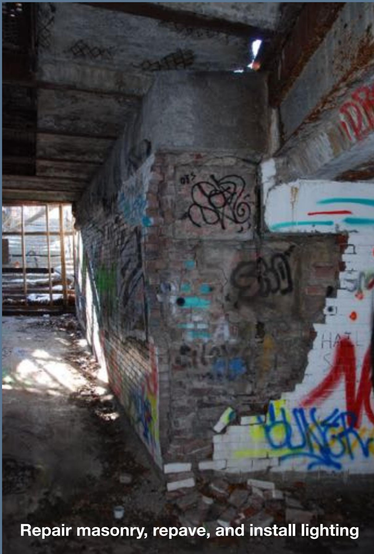
Repair masonry, repave, and install lighting
